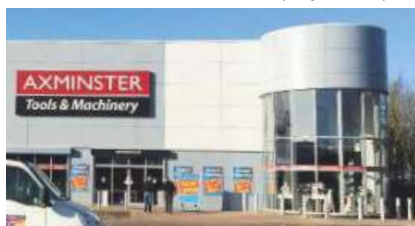
Axminster's North Shields store, which opened in March this year
